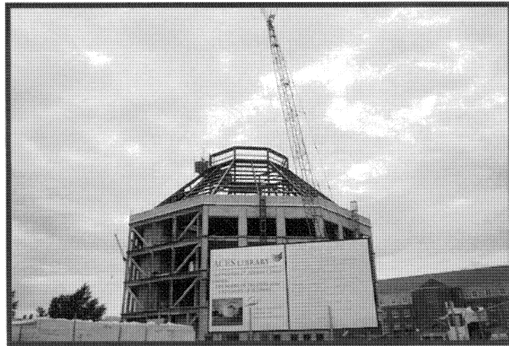
The new ACES Library under construction.
